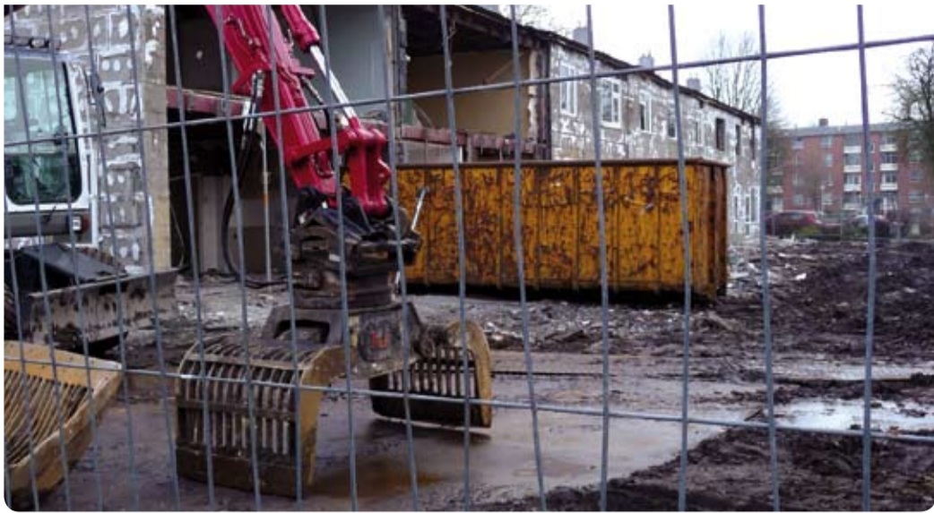
De sloop is in volle gang
